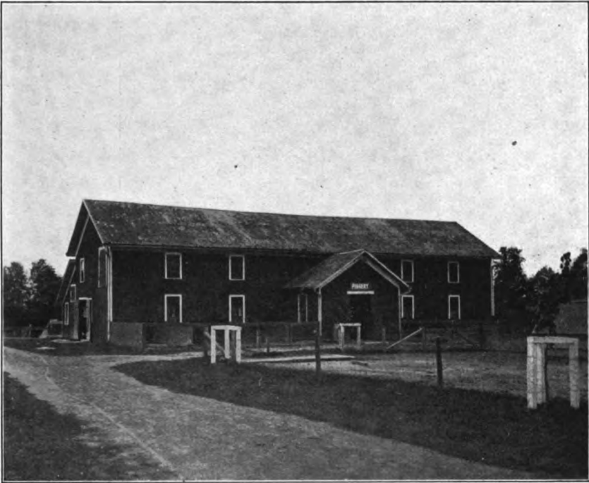
Piggery built by Dr. Miles, twice moved.
